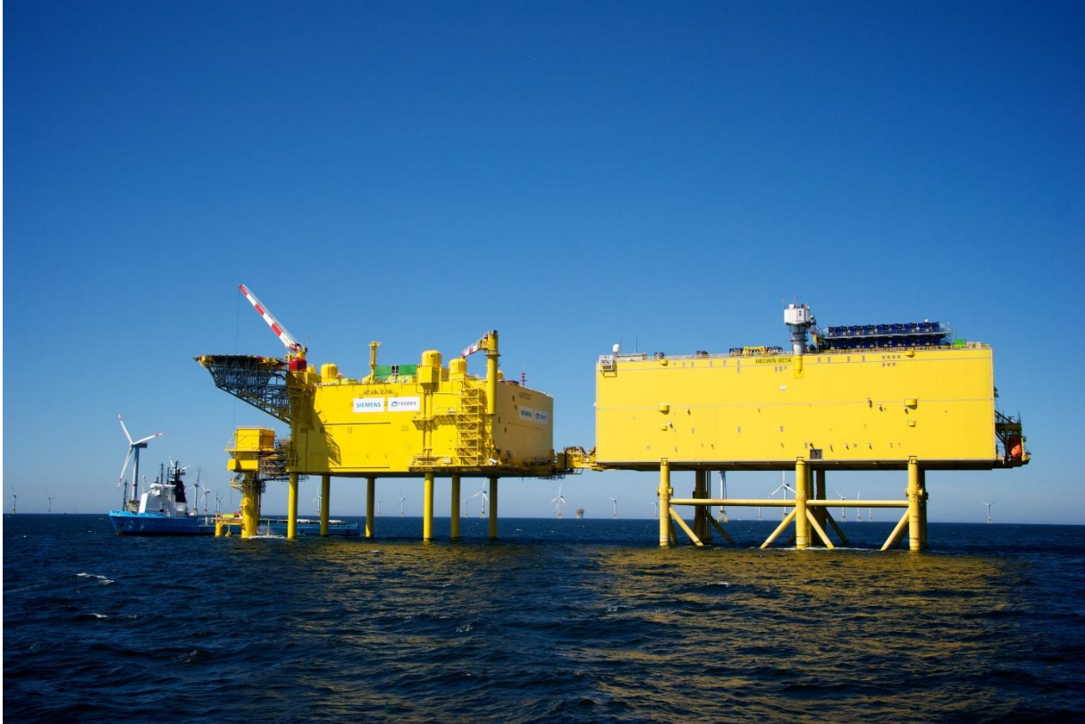
Figure 2 - Extinguishing systems must function correctly to provide optimum protection against fires! – Structures located in the North Sea are no exception. HelWin beta Copyright TenneT
